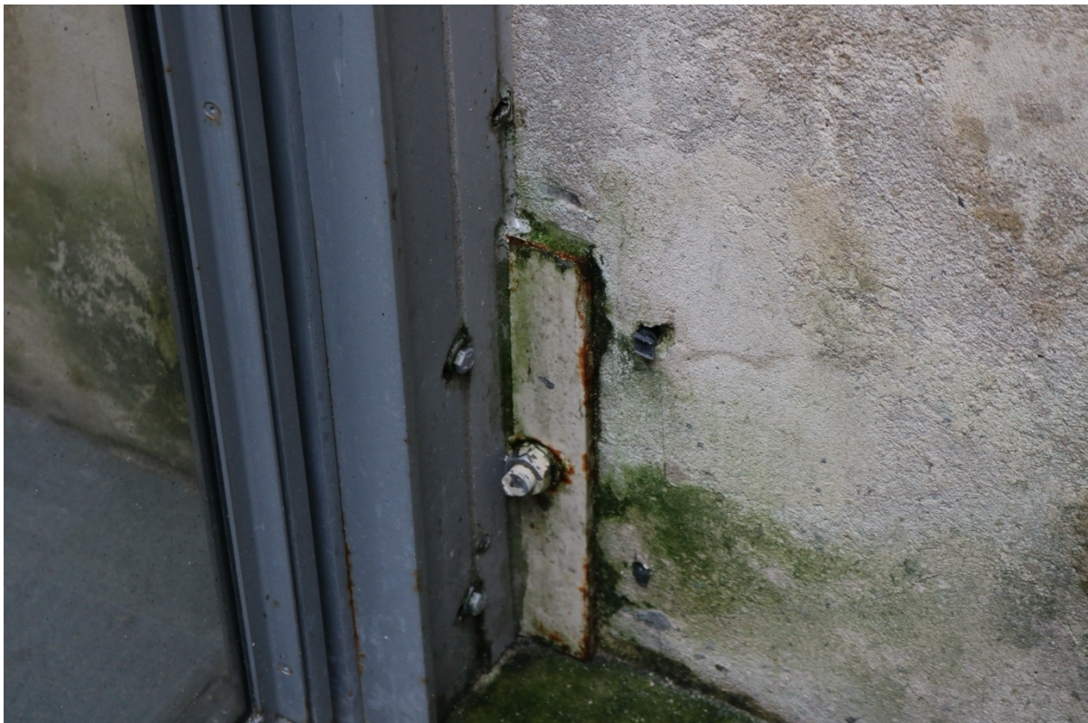
Figure 2.3 - Junction detail: grey aluminium frame meeting masonry wall, colour-matched steel plate. Author's photograph, December 2025.
